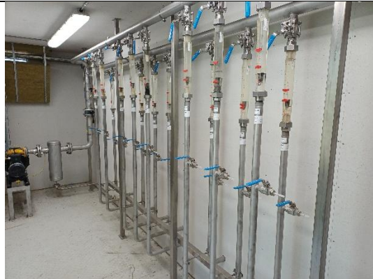
Deponi III. Kig ind i container for biocoverstyring
