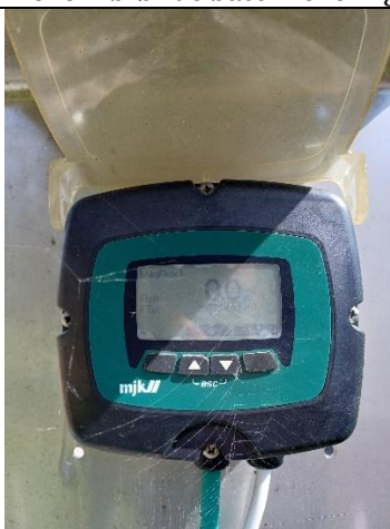
Deponi III. Flowmåler for pumpebrønd G
