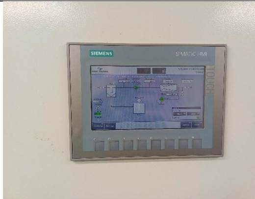
Deponi III. Overvågning for biocover/gas.
