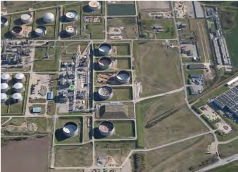
Figure 1-1: Fredericia Oil Terminal 12
