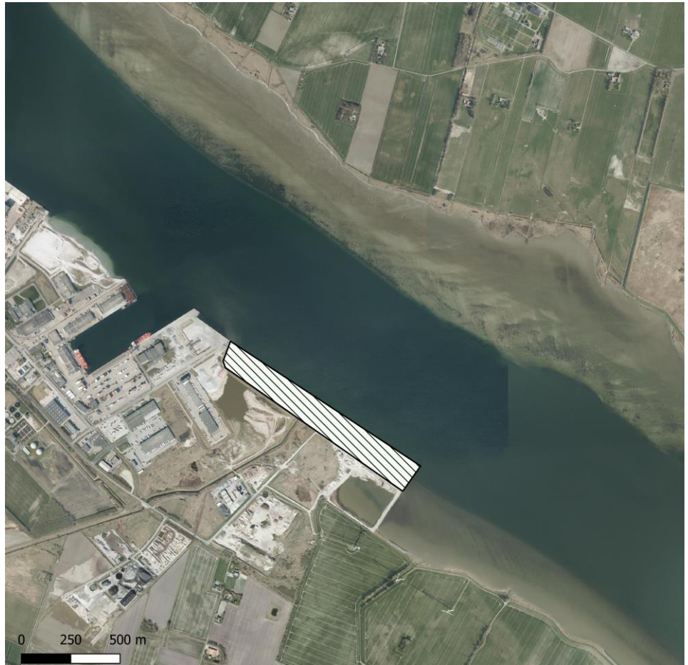
Figure 1: Quay Wall Extension
