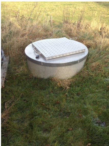
Figur 4 Monitoringsbrønd M8 (SØ for deponiet)
