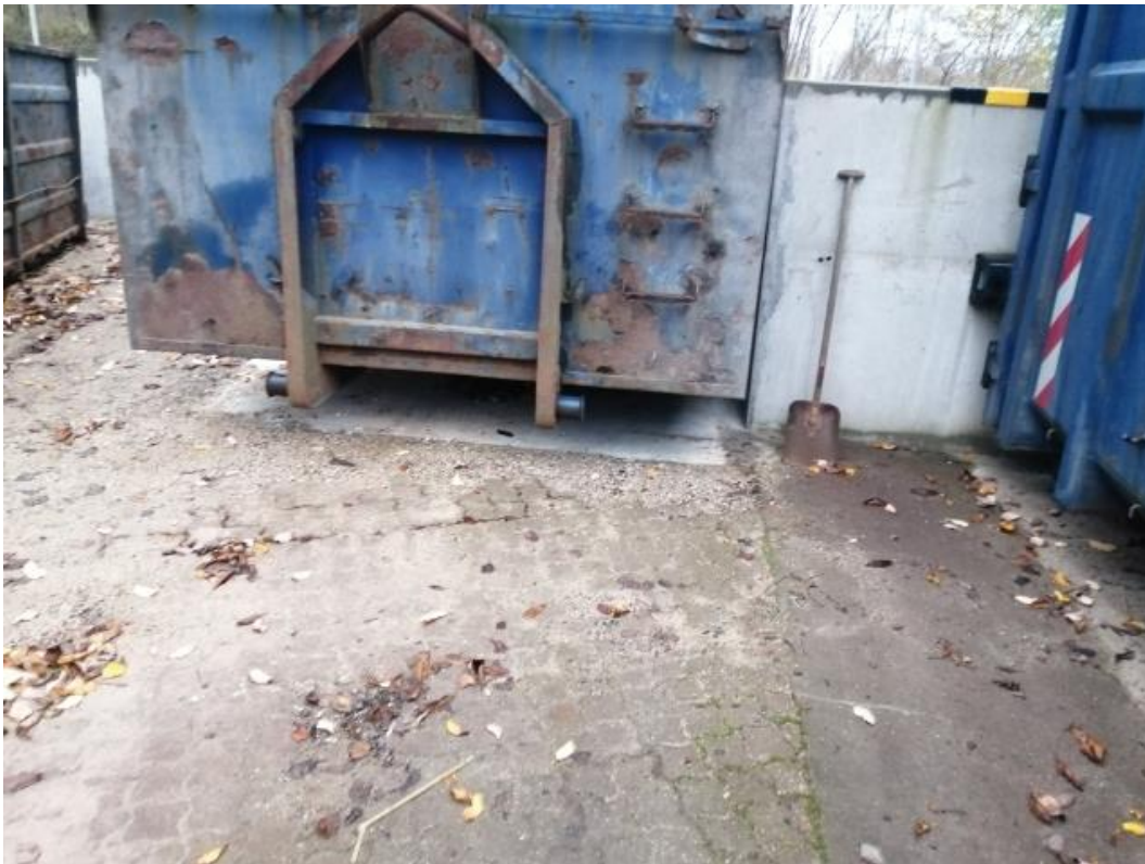
Ny belægning under ny metalcontainer.
