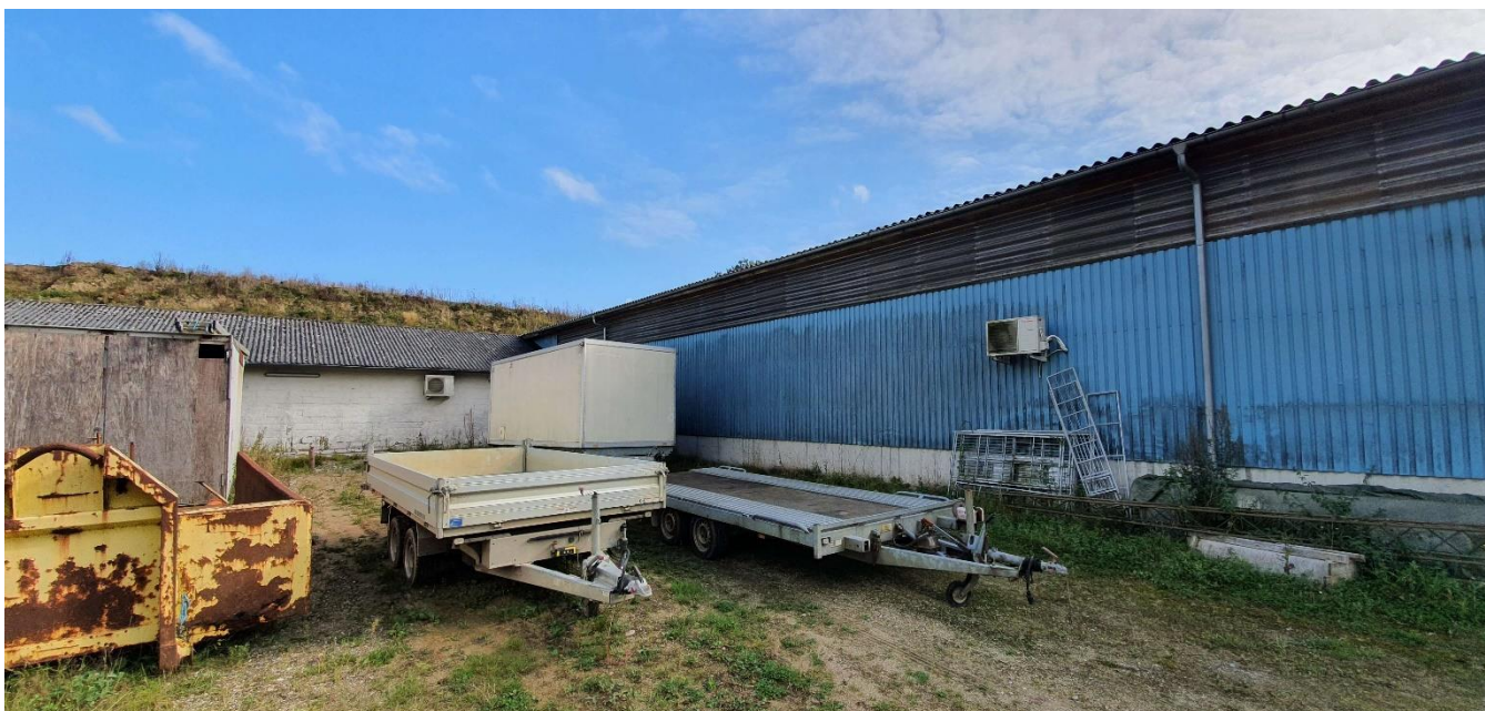
Her ses de to luft/luft varmepumper.
