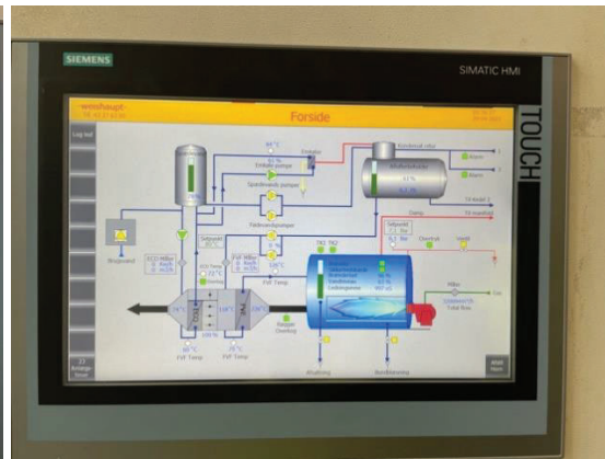
TH. Drift 6 tons kedel.
