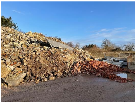
Beton, ca. 7-8.000 tons
