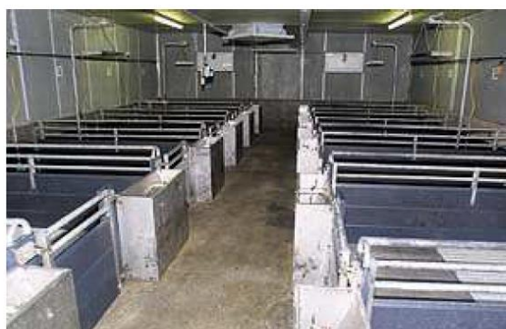
Figure 1: interior view of the control room
