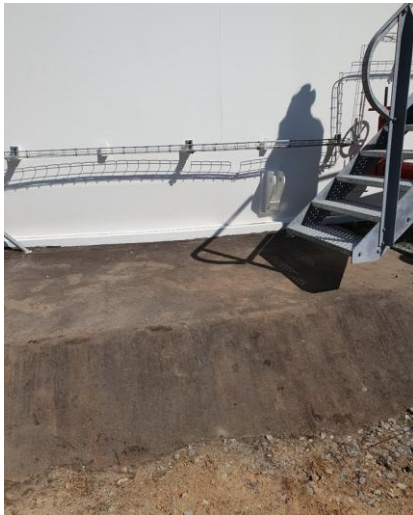
Foto 1: Ny tankpude under tank T23
