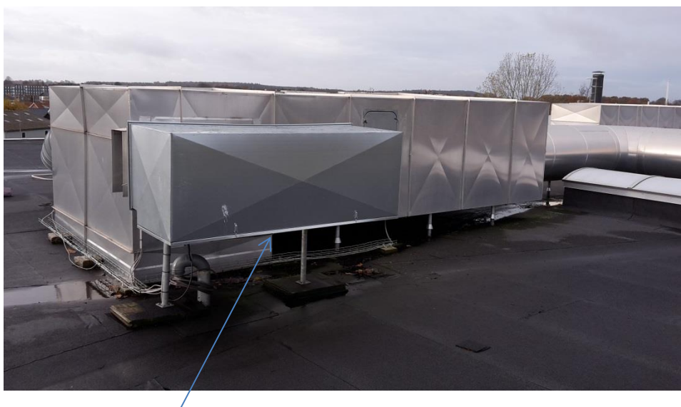
Indsugning ventilation
