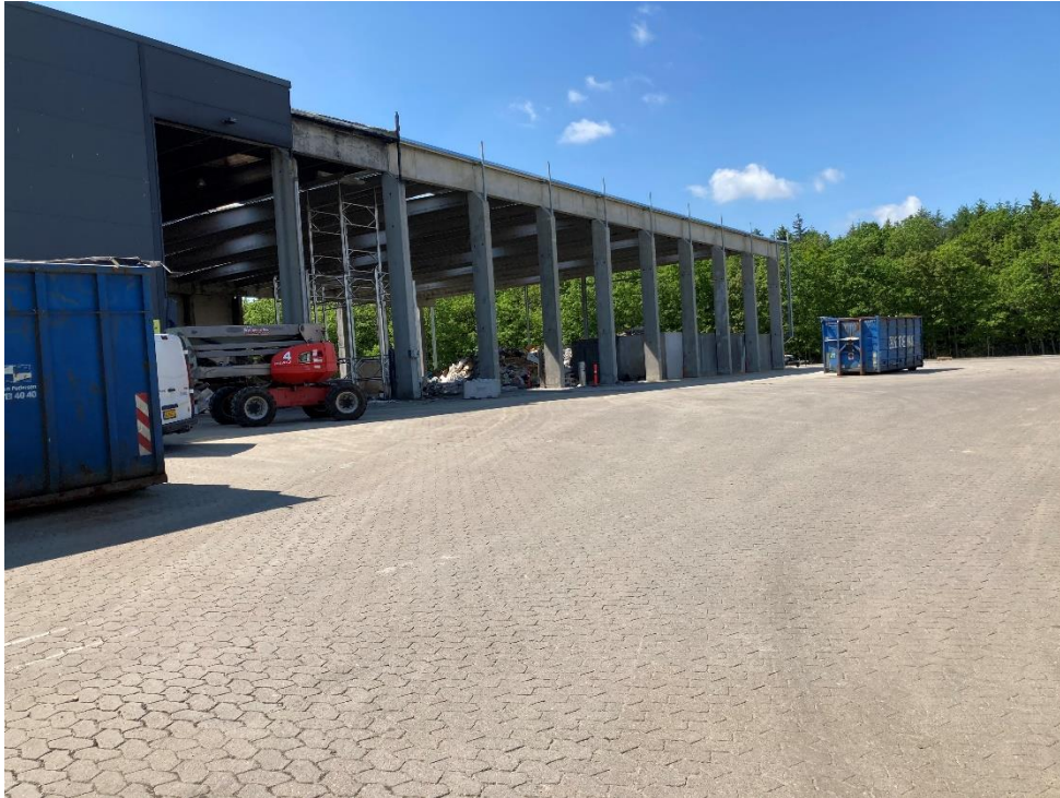
Hal under renovering
