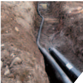
Reused for backfilling
