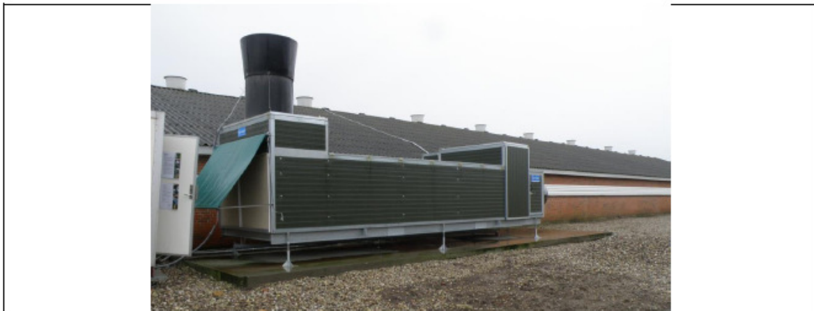
Figure 1. Picture of the Agro Clima Unit situated outside the test broiler section. Ventilation air to and from the broiler house are drawn through the Agro Clima Unit by a counter current principle to utilise the heat content of ventilation air to heat up inflowing air.
