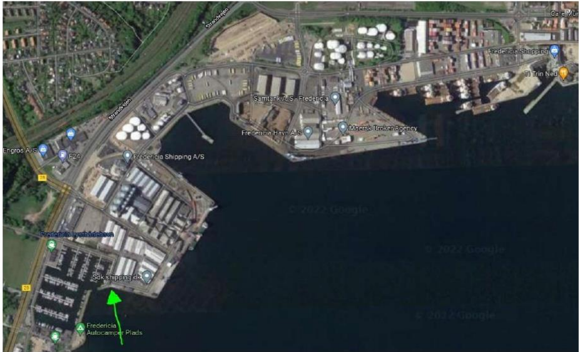
Figure 2: Planned location of the test system indicated with the green arrow (source: ADP A/S)
