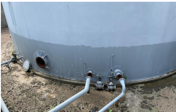
Tank 1, afmonterede ventiler
