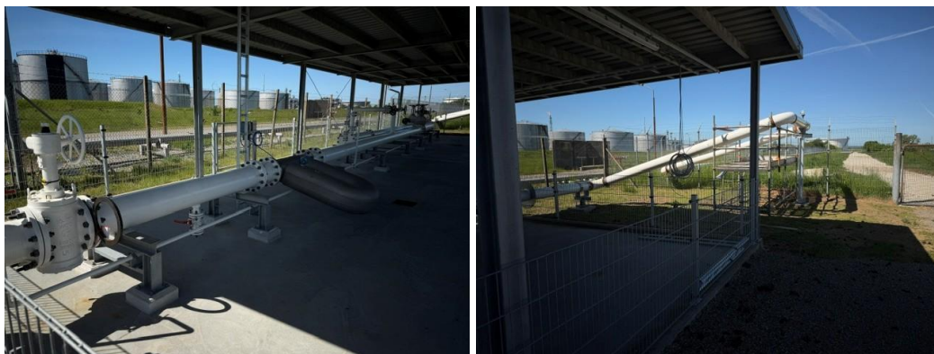
Figur 8. Tie-in punkt for pipeline
